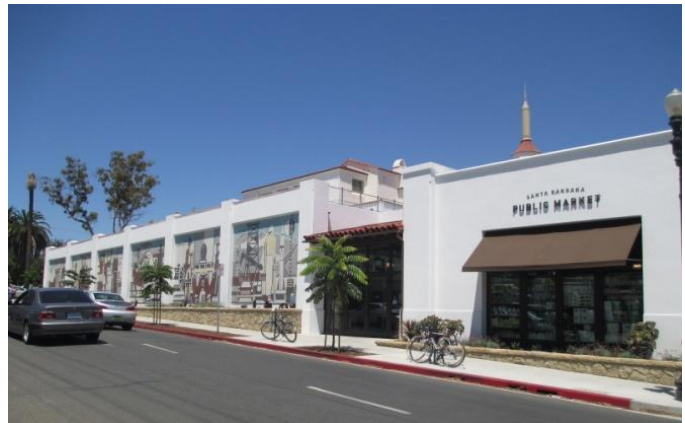
Above and below: Views of the Knowles mural in their new location and setting on the West Elevation of the Mediterranean Style new Public Market Building facing Chapala Street, photos taken August 2014
