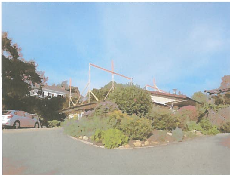
V2 View from driveway looking Northeast at house
