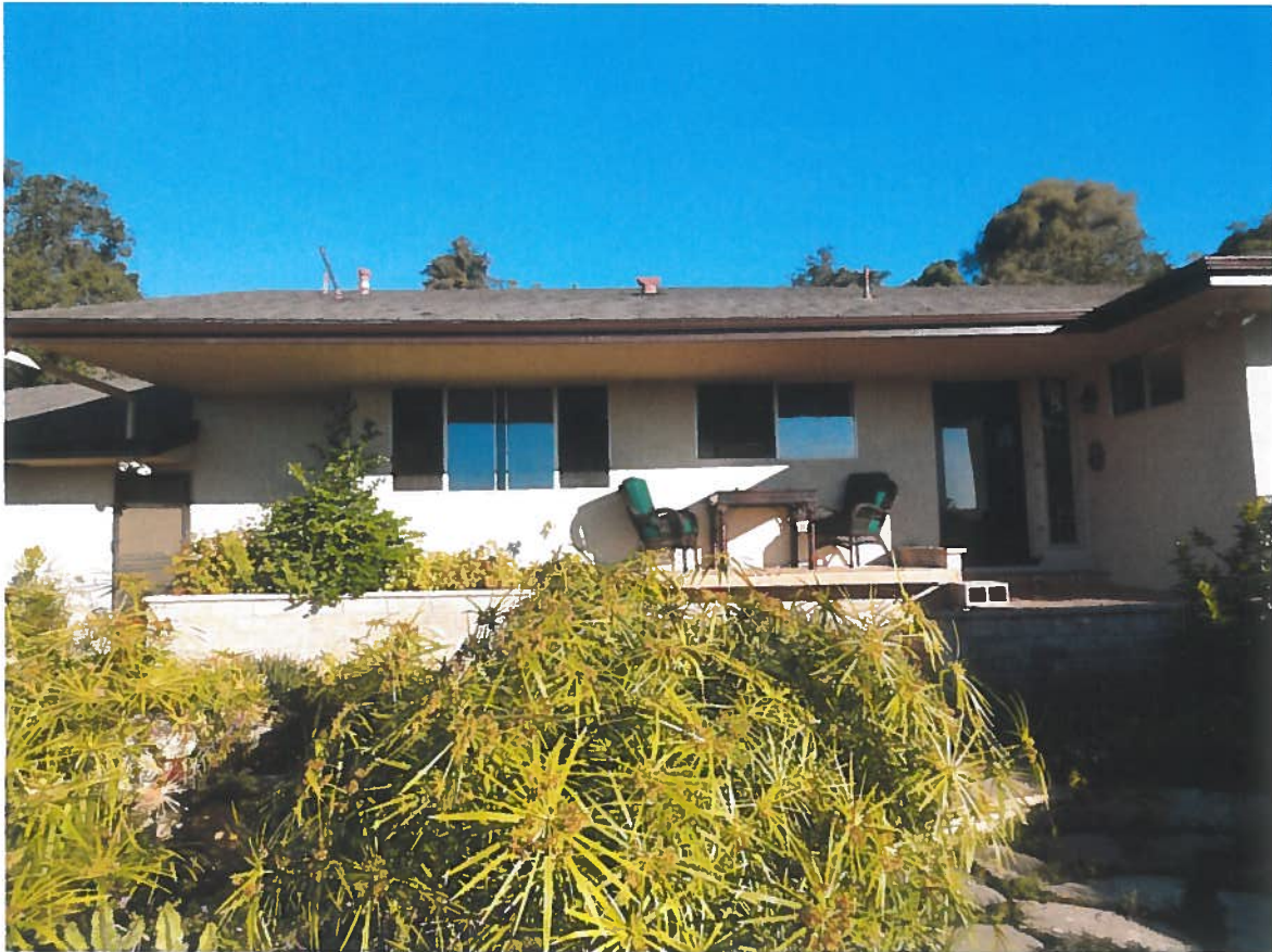
View from South looking at existing residence main entrance
