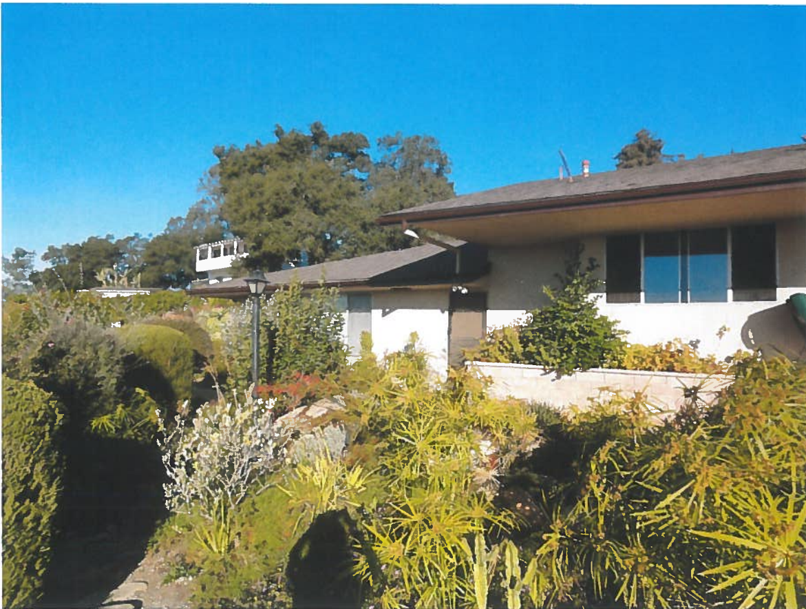
View from South looking at existing garage
